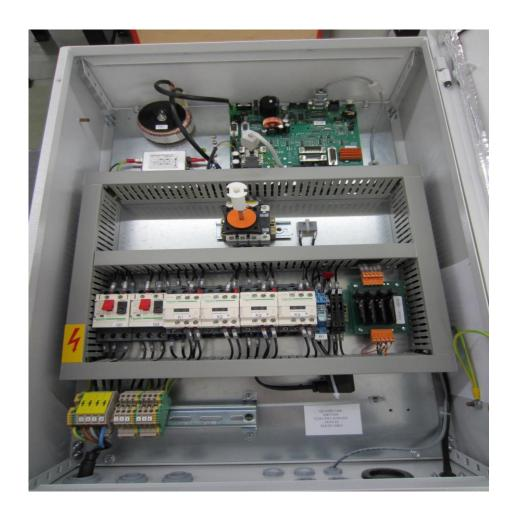
Connect the external power supply 400V AC from the interlocked socket terminals marked R-S-T-N and ground and connect the motors of the bench to the power module (pictured below).
