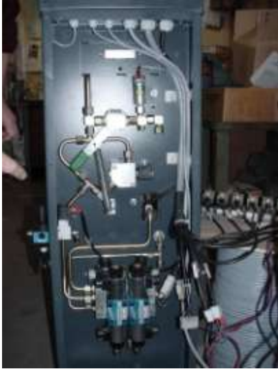
Pic 13: Connection of hydraulic hoses in command unit
