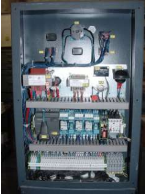
Pic.15 Electrical parts in command unit
